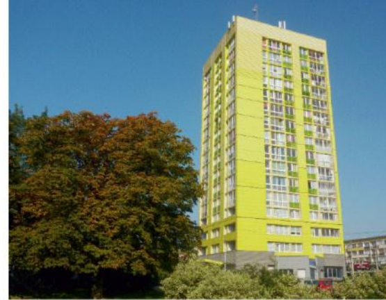
Rainscreen cladding, Cassette system
